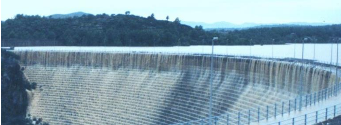
Figure 1. Overtopping of the dam crest.
