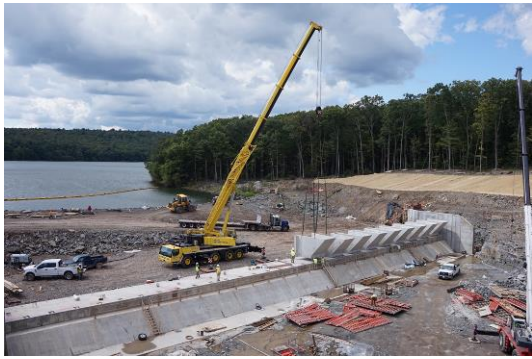
Fig. 14 Fusegate Installation at Pikes Creek
