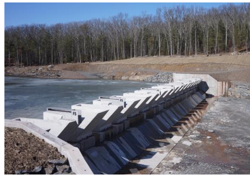
Fig. 15 Completed Fusegate System at Pikes Creek
