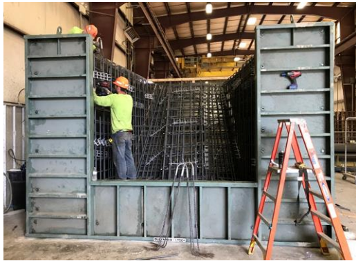
Fig. 11 Custom-made formwork and steel placement F..
