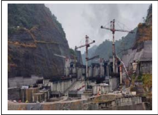
View of Dam from D/s end
