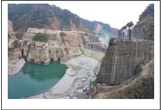
View of Diversion Tunnel, Dam and Intake
