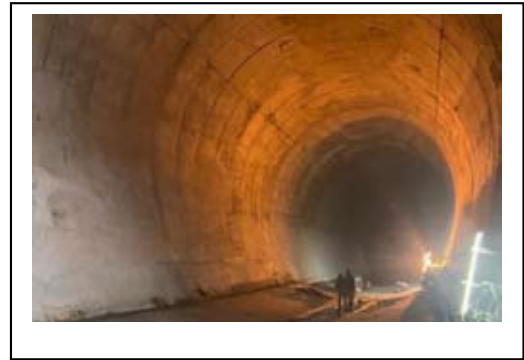
Head Race Tunnel
