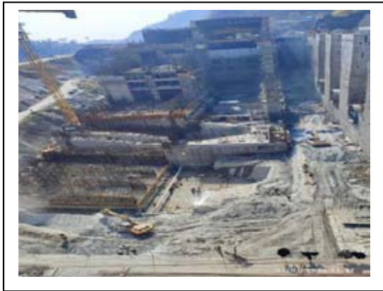
View of Power House
