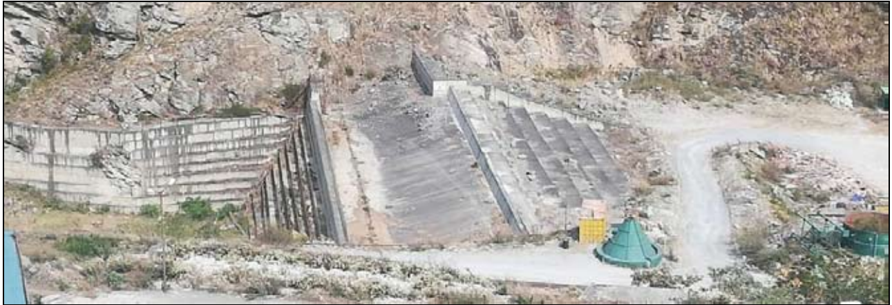
Fig. 9 : Constructed coffer dam, top view from right bank
