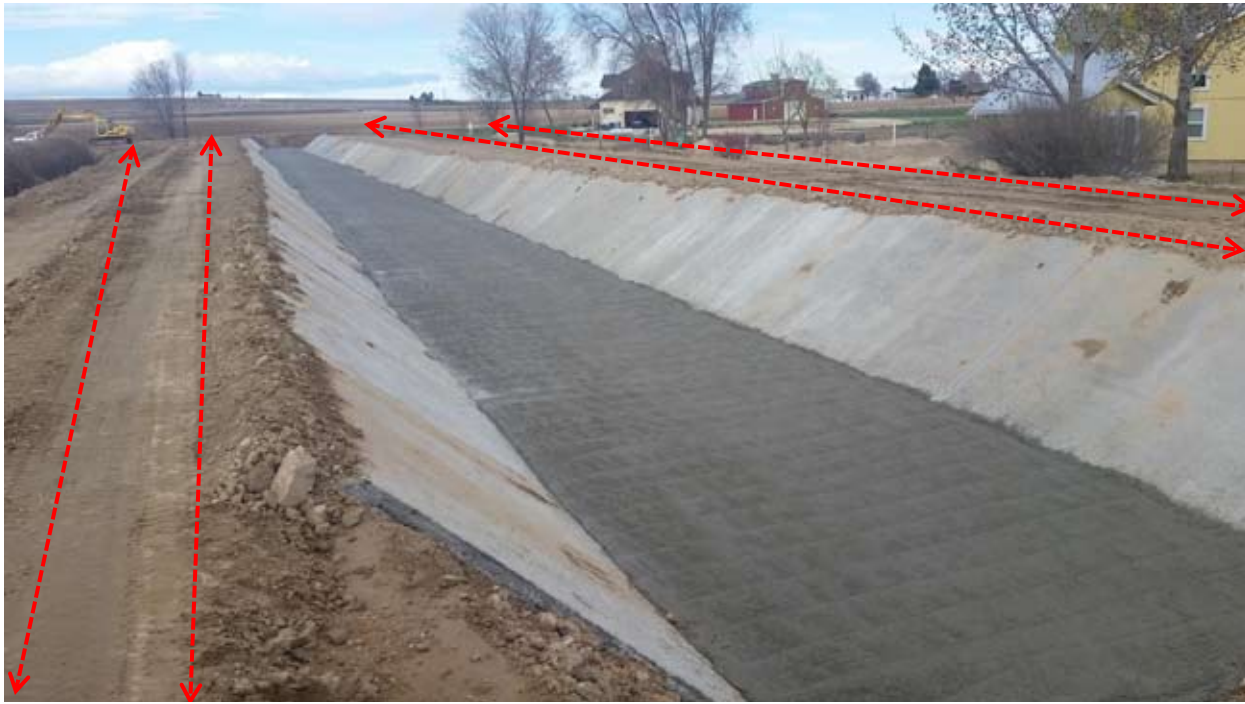
Fig. 14 : Indicative ERI and SP Profiles Along a Lined Canal
