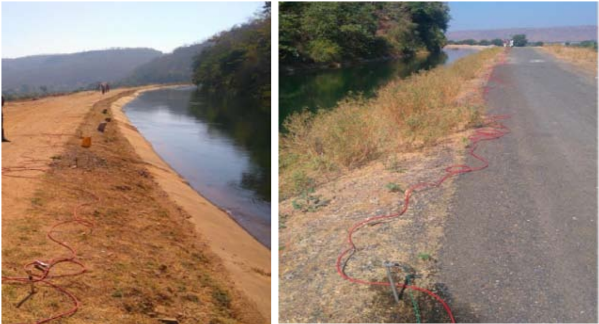
Fig. 15 : ERI Profiles for canal seepage studies in Gujarat
