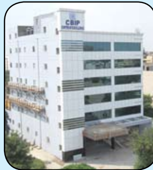
CBIP Centre of Excellence at Gurgaon (2013 onwards) Sector 32, Plot No. 21
