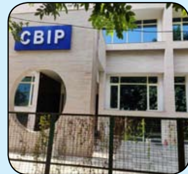
CBIP Centre of Excellence at Gurgaon (2020 onwards) Sector 32, Plot No. 09
